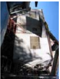
View of Building D - Trailer Office
